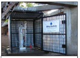
The SkyHydrant is secured in a steel enclosure to ensure that this valuable equipment is safe and ready for use
