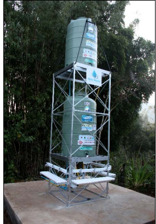
The SkyJuice SkyTower completes the safe water system providing self closing taps, water troughs and hand wash station.
