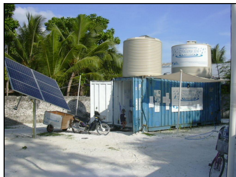
Figure 9: Solco "Meeru Fen" Water Factory, Maldives Containerised RO plant including delivery service
