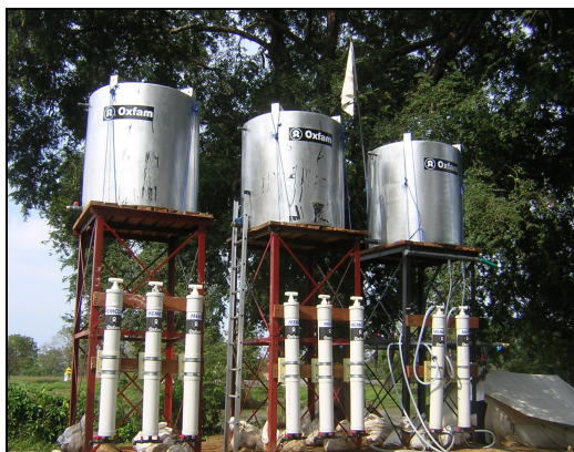
Figure 10: Installation undertaken in Sri Lanka –IOM IDP camp installation (100,000 L/d capacity)
