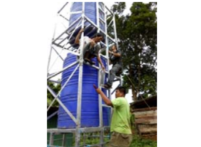
Fixing the frame and tightening the screws
