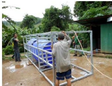
Getting ready for the LIFT!
