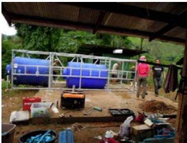
Fitted the frame and tank together
