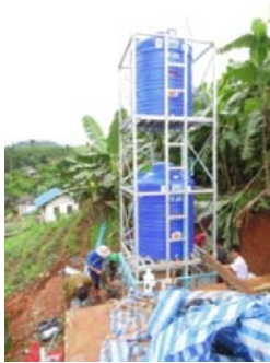
Fitting the frame and tank together
