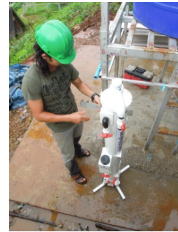
Fixing the frame and SkyHydrant to the concrete slab
