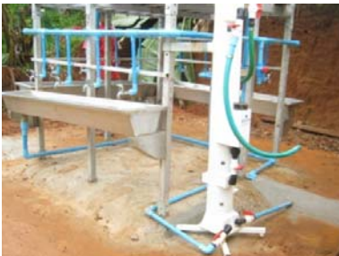
Fitting the pipes to the water source
