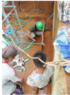
Getting ready for the LIFT!
