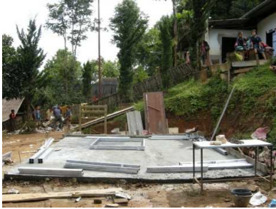
The foundation has been laid.
