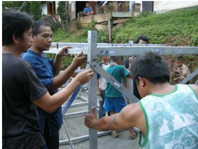
Involving community members in the installation process
