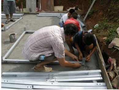
Starting the installation process.
